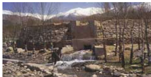
Fig. 6. Zings are used to collect snow melted water
